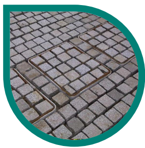
Block Paved Install
